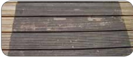
Fig. 24: Te dunne laag Nylo bruggencoating
